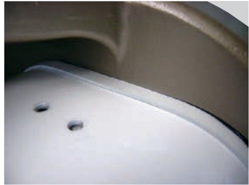
Cover top temporarily removed
